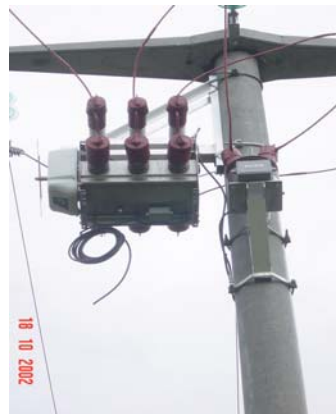
Figure 4 - New generation of pole mounted switch disconnector for remote control
